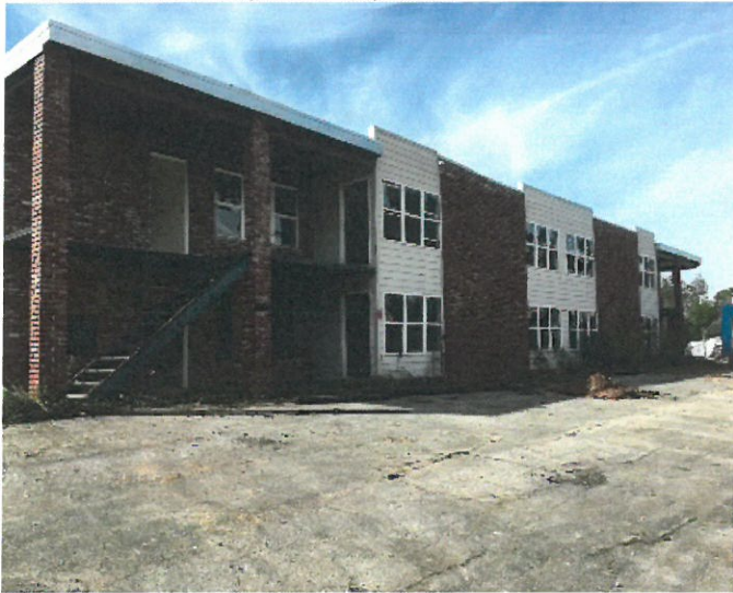
12 CENTER PL N (BLDG 12) 35204
