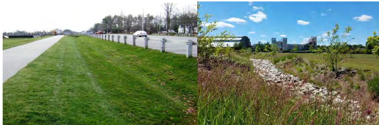
Vegetated BMPs can look like mowed grass, such as this vegetated swale on the left, or like landscaping, such as this urban bioretention area on the right.
