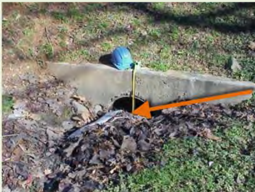
Debris and leaf litter are blocking this inlet. Remove this material to allow water to enter the inlet.
