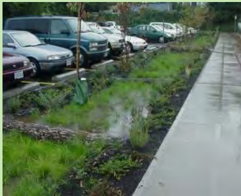
Urban Bioretention Area after a Rain
