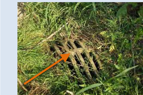
Grass has grown over this inlet and should be cut back to allow water to enter the inlet.
