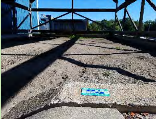
Figure 6.18.1. Sand Filter
