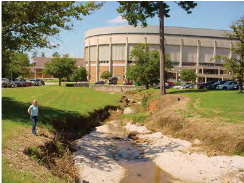
Figure 1-6. Parkerson Mill Creek Erosion, Auburn AL (Source: Storm Water Solutions Newsletter, Feb. 6, 2017 )
