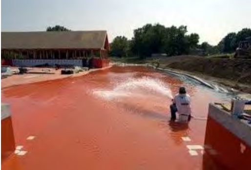
Figure 6.10.3. Flood Testing the Waterproofing Layer
