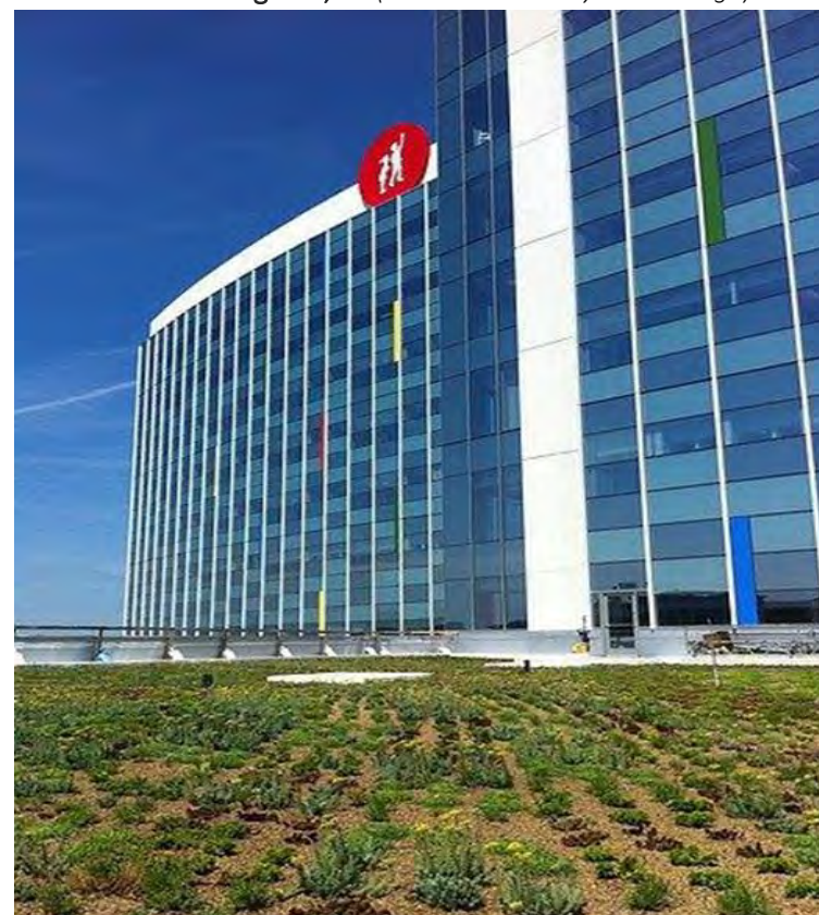
Figure 4-5. Intrinsic GIP (Green Roof) at Children’s Hospital in Birmingham, AL (Source: Macknally Land Design)
