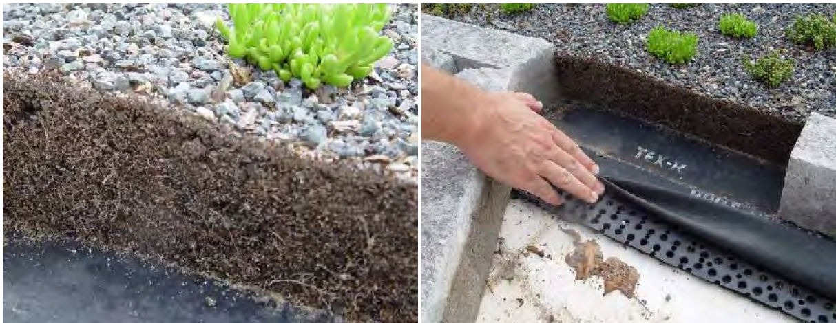
Figure 6.10.2. Vegetated Roof Cross-Sections (Source: B. Hunt, NCSU)
