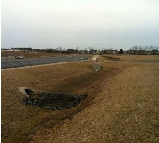
Figure 6.14.1. Example of Dry Detention Pond
