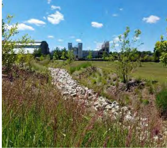
Figure 6.5.1. Example of Dry Water Quality Swale
