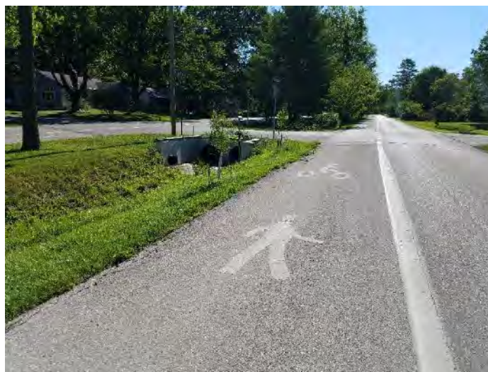
Figure 6.5.2. Example of Grass Channel along ROW
