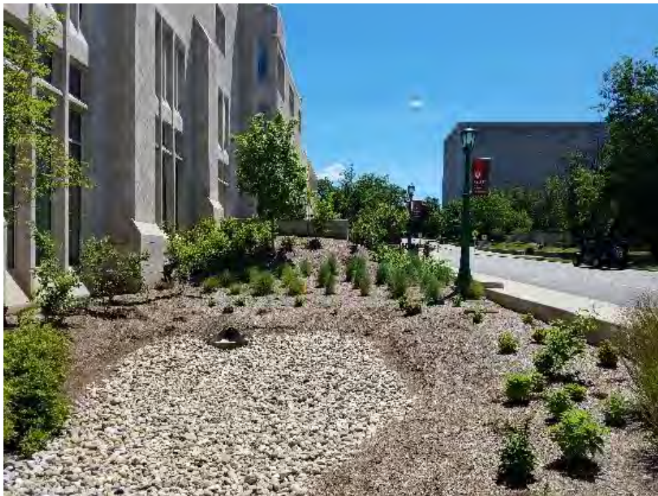
Figure 6.4.4. Example Urban Bioretention Area
