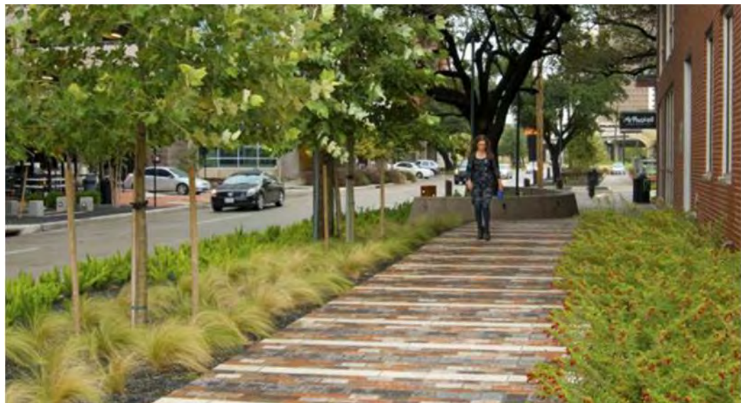
Bottom: A complete street was designed for the reconstruction of Bagby Street in Houston TX. The street includes numerous features for storm water management. (Credit: Design Workshop)
