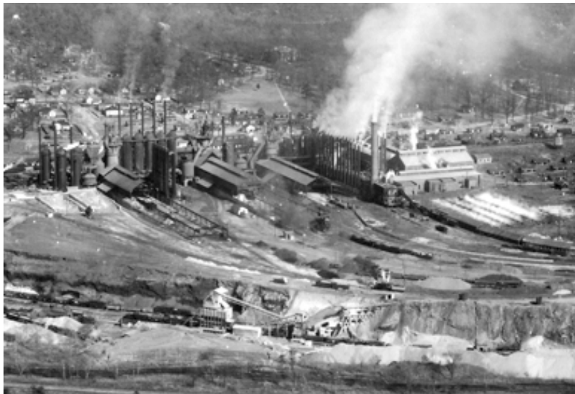
Figure 1-9. Woodward Iron Company, Founded in 1881 (Source: encyclopediaofalabama.org )
