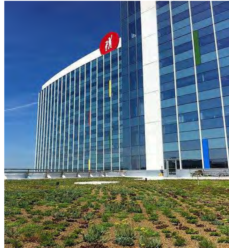
Figure 1-21. Green Roof in Benjamin Russell Hospital for Children in Birmingham, AL (Source: Macknally Land Design)
