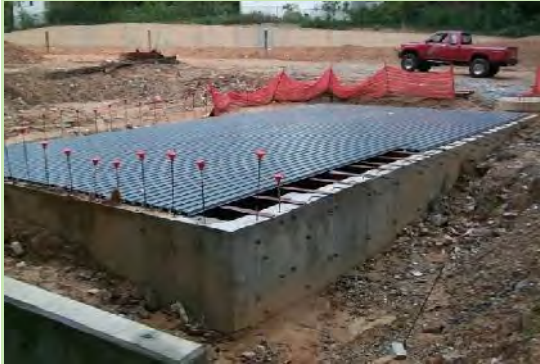
Figure 6.17.1. Underground Detention Construction
