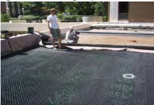
Figure 6.10.4. Drainage Layer Installation
