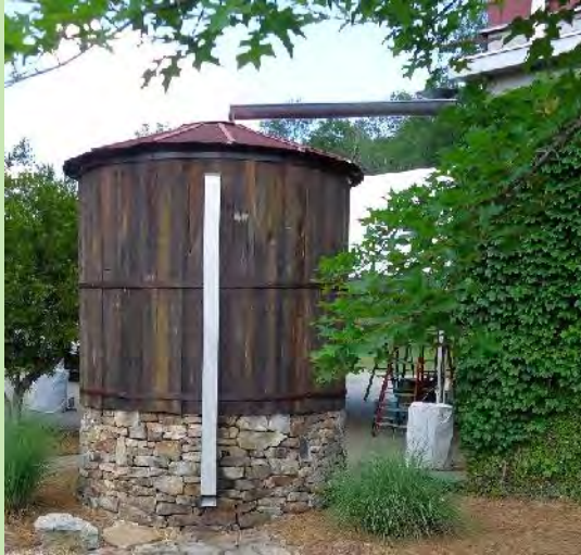
Figure 6.13.1. Cistern at Stewart Perry Construction, Birmingham, AL
