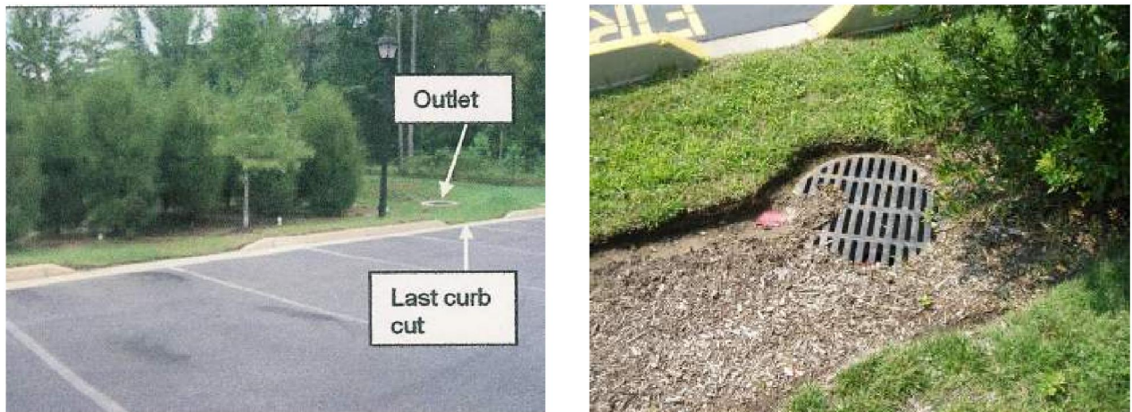
Figure 6.3.4. Examples of Short-Circuiting at Bioretention Facilities (Source: VADCR, 2010)
