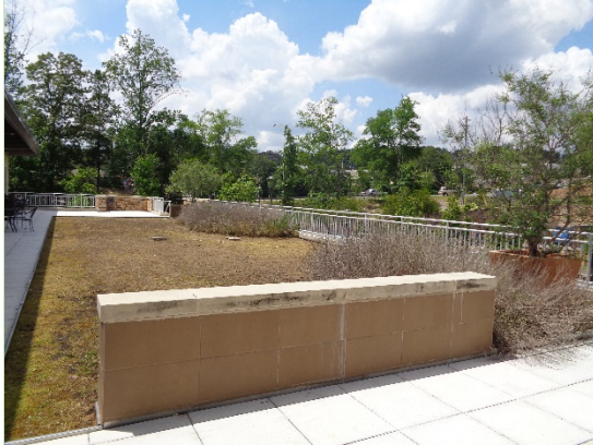
Figure 6.10.1. Vestavia Hills Public Library Green Roof in Birmingham, AL
