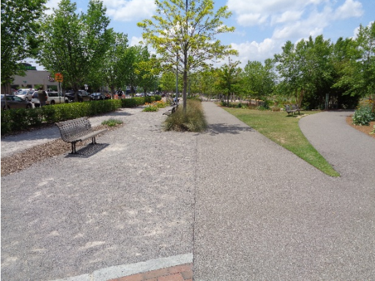
Figure 6.11.1. Permeable Pavement in Railroad Park in Birmingham, AL
