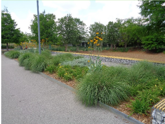
Figure 6.12.1. Infiltration Area at Railroad Park, Birmingham, AL
