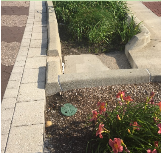
Figure 6.4.1. Urban Bioretention Area along Indianapolis, IN Cultural Trail
