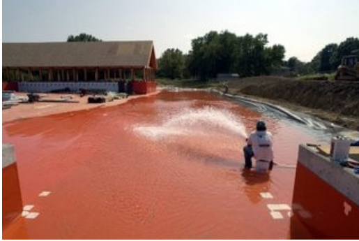
Figure 6.10.3. Flood Testing the Waterproofing Layer
