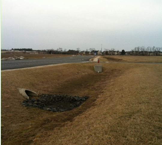
Figure 6.14.1. Example of Dry Detention Pond
