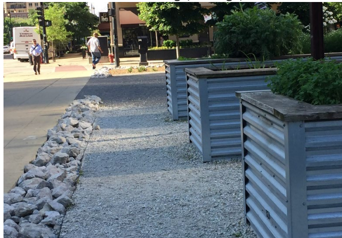
Figure 6.12.2. Infiltration Trench in Papermaker’s Garden, Columbia College, Chicago, IL
