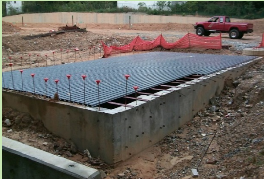
Figure 6.17.1. Underground Detention Construction
