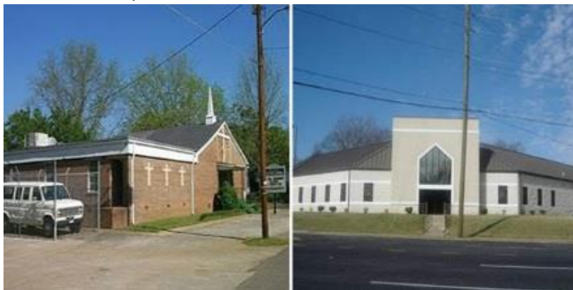
Figure 1-11. St. James Baptist Christian Center Before / After Acquisition and Relocation (Source: floodsciencecenter.org)
