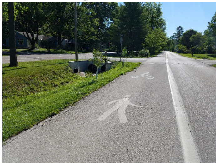
Figure 6.5.2. Example of Grass Channel along ROW
