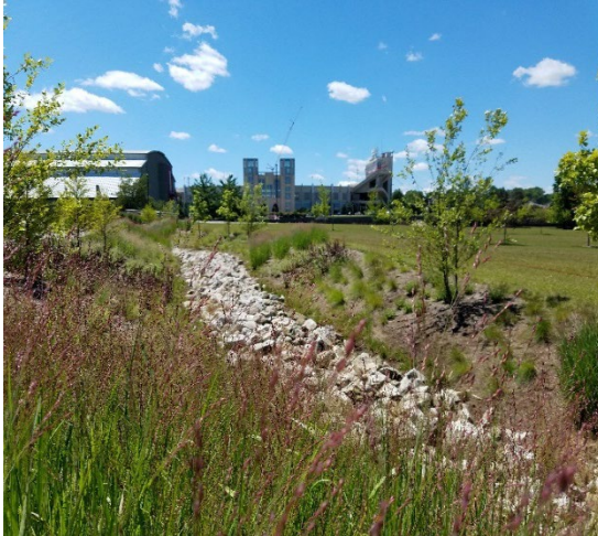
Figure 6.5.1. Example of Dry Water Quality Swale
