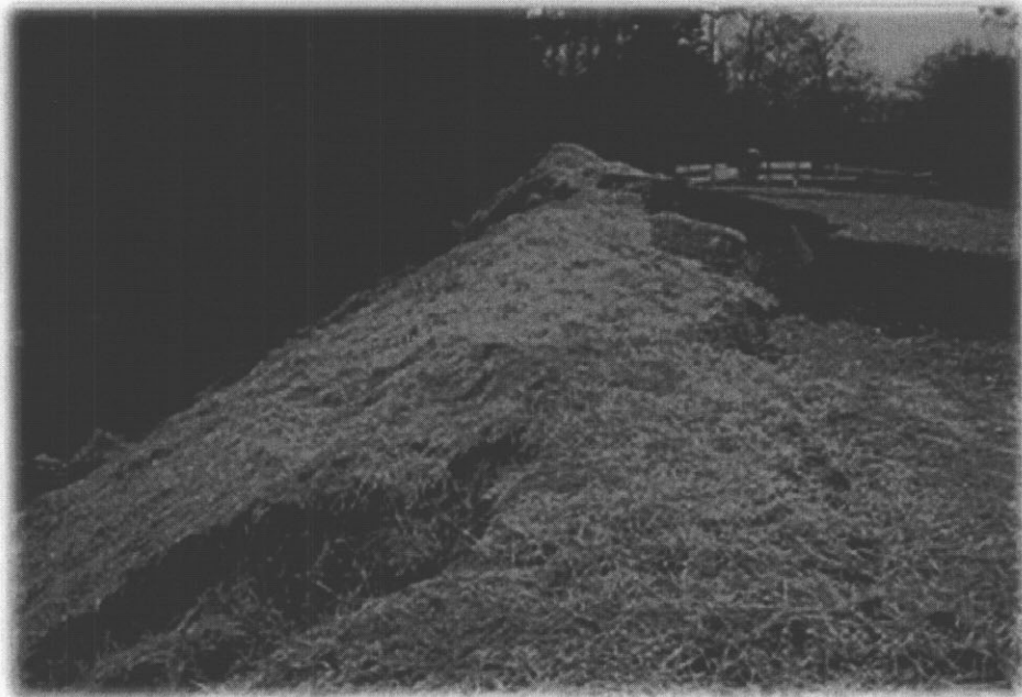
Straw being used to reduce erosion
