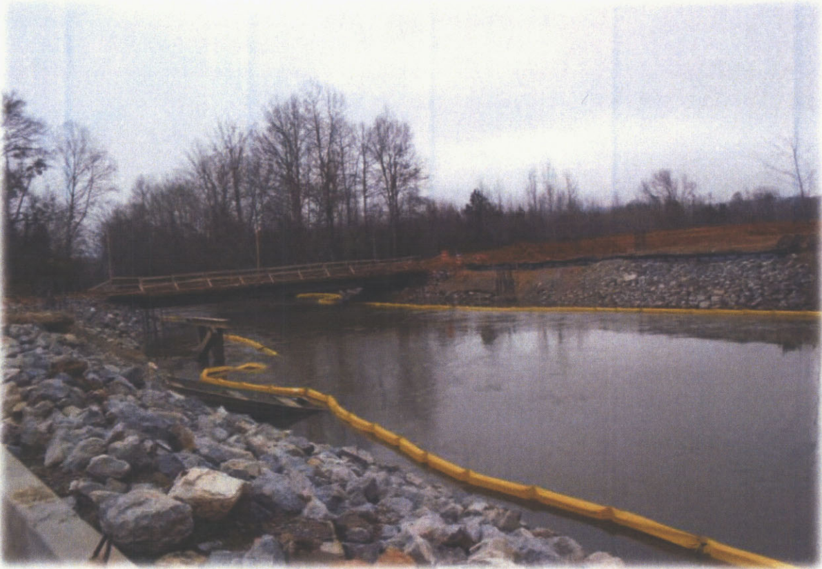
The combined efforts of the turbidity curtain and other BMPs
