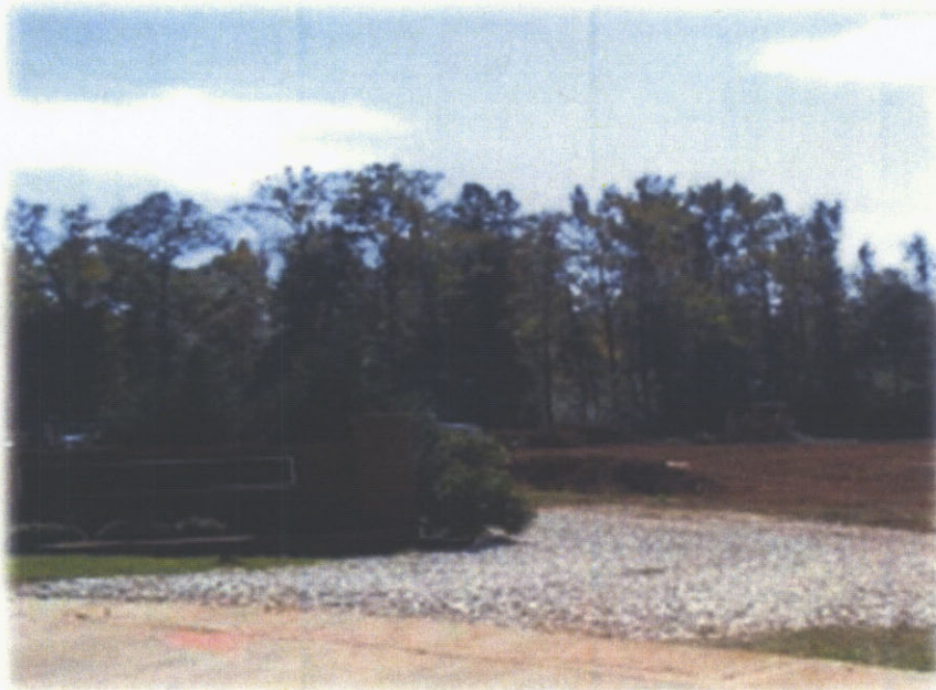
Construction Exit Pad
