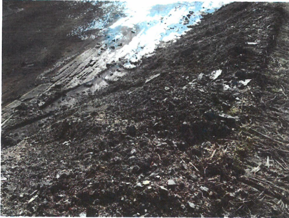
Disturbed Creek Banks
