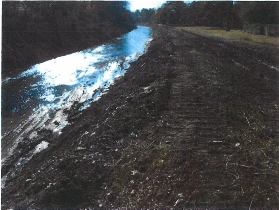
Disturbed Creek Banks
