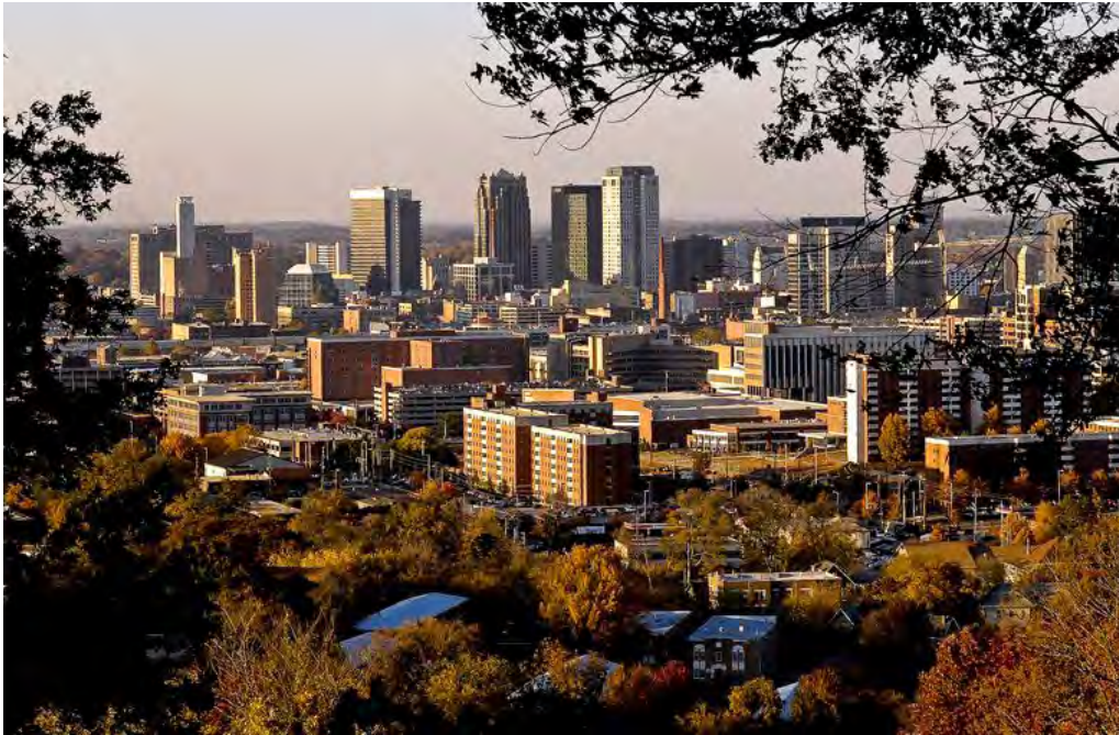
Figure 65: University of Alabama at Birmingham
