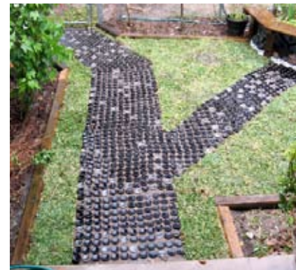
Bottles used as construction material for a pathway
